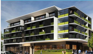
FORTUNE HIGHWAY - II Next to Fortune Highway, Jain Pete, Moodbidri
